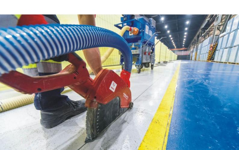
Expansion joints found in industrial floors are subject to natural degradation under the influence of operating loads and the work of the floor slab. The method of expansion joint repair depends on the type and degree of damage.
