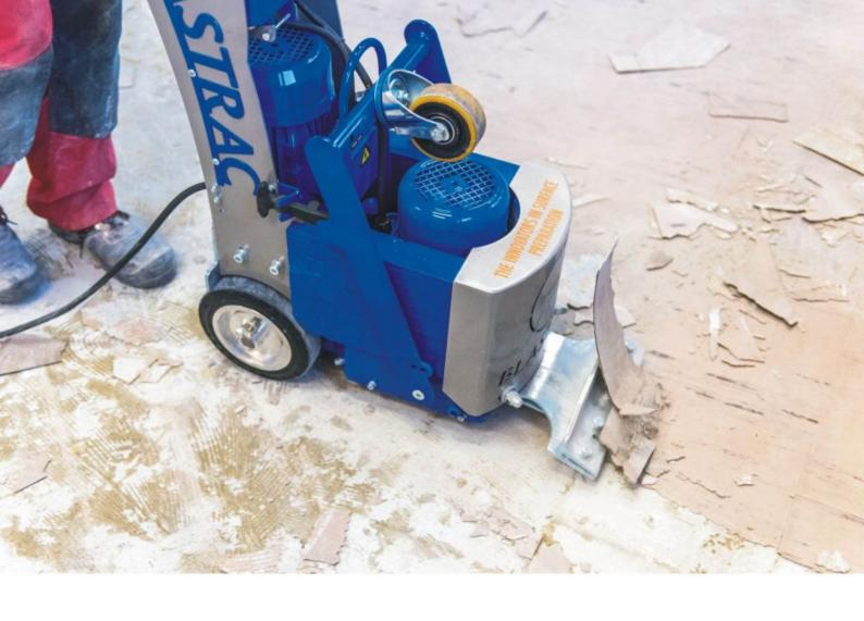
Apart from the highest work efficiency, the machineassisted tile stripping method reduces the nuisance of traditional methods, such as manual jackhammering. The substrate is not damaged during work and percussive operations are kept to a minimum.
