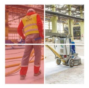
Apart from an impressive decorative effect, the surface is characterized by high resistance to abrasion and low maintenance costs thanks to which the polished concrete can remain in perfect condition for many years.
